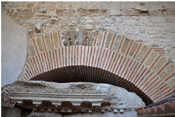
Fig. 5. Peristyle, relieving arch above the portal leading into the Vestibule after restoration (photo: Croatian Conservation Institute)
