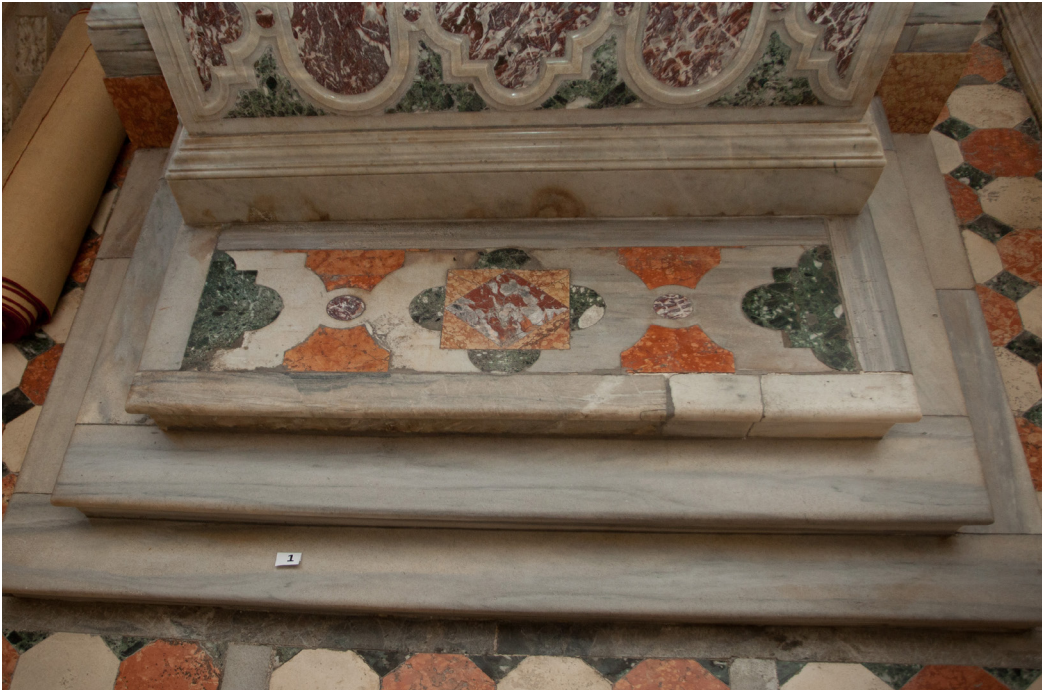
Fig. 2. Steps and the predella (platform) of the altar (photo: Z. Sunko)
