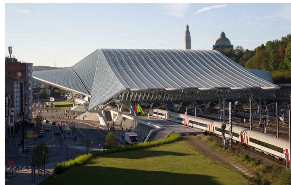
Liege-Guillemins station, Santiago Calatrava, Liege, Belgija
