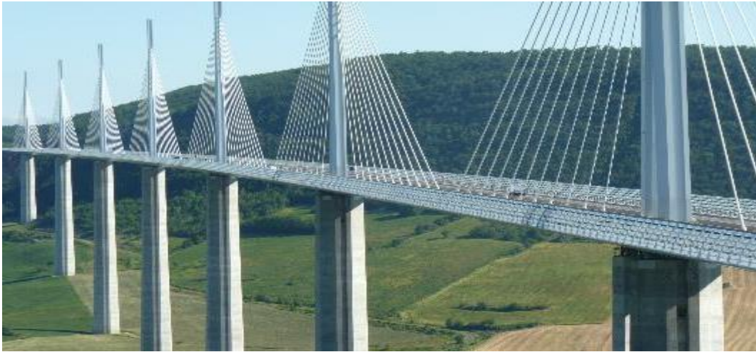
Figure 2.12- Viaduct de Millau ( http://circuitosvip.blogspot.pt/2015/01/viaduto-de-millau-franca.html , 2015)
