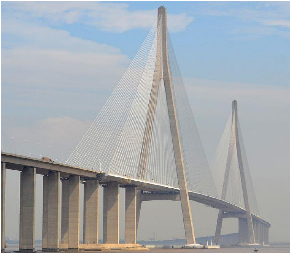
Figure 2.6 – Sutong Bridge (Wikipedia, 2015)
