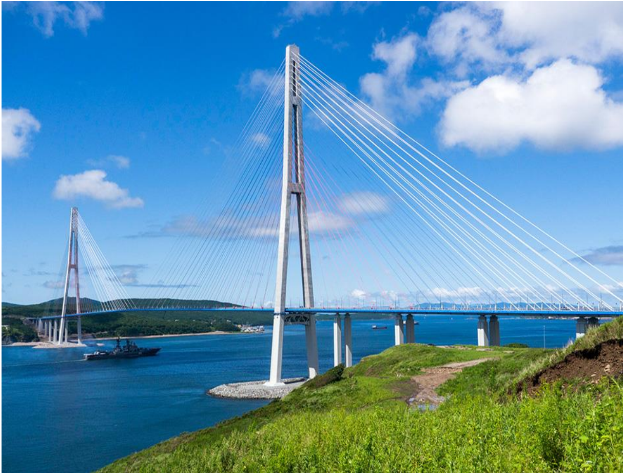
Figure 2.7 – Russky Bridge ( http://rusbridge.net/ , 2015)
