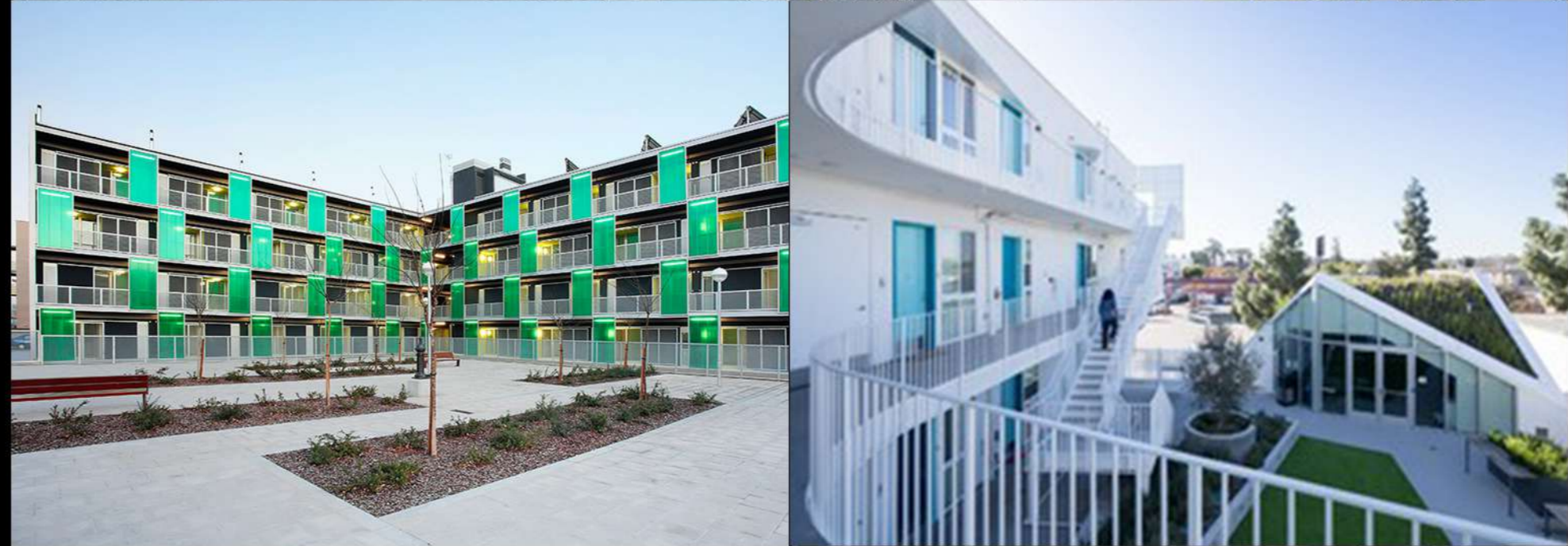
44-units social housing in Pardinyes Coll-Leclerc Arquitectos Lleida, Španjolska_2010.
