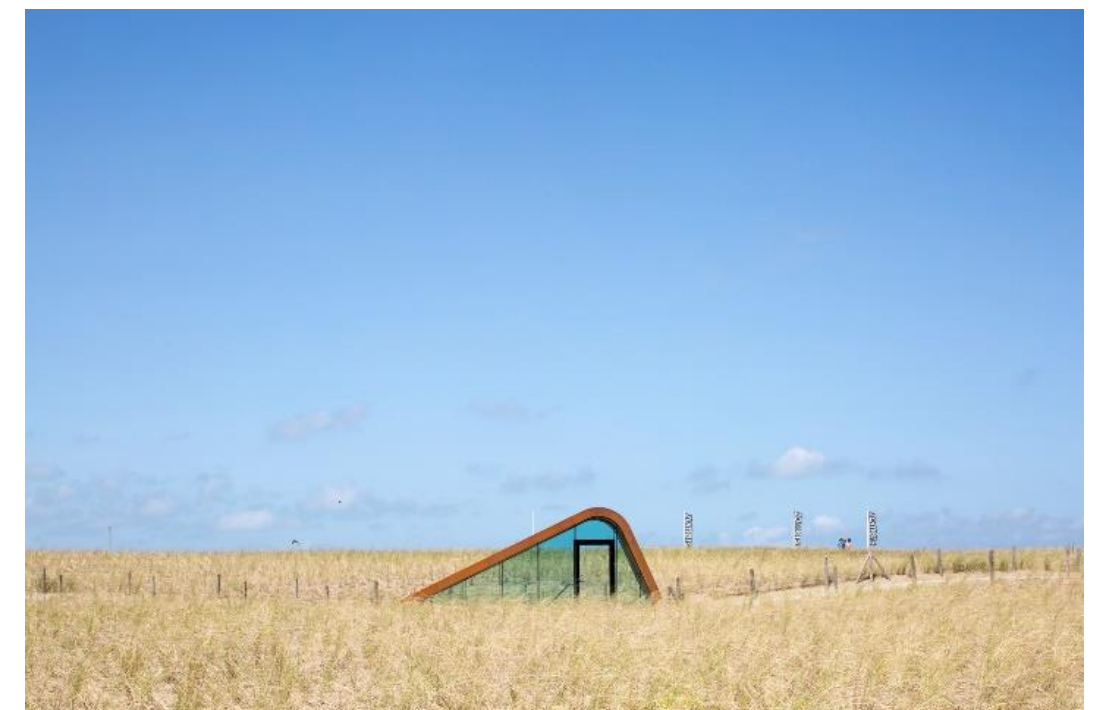
Underground parking - Royal HaskoningDHV, Nizozemska, 2016
