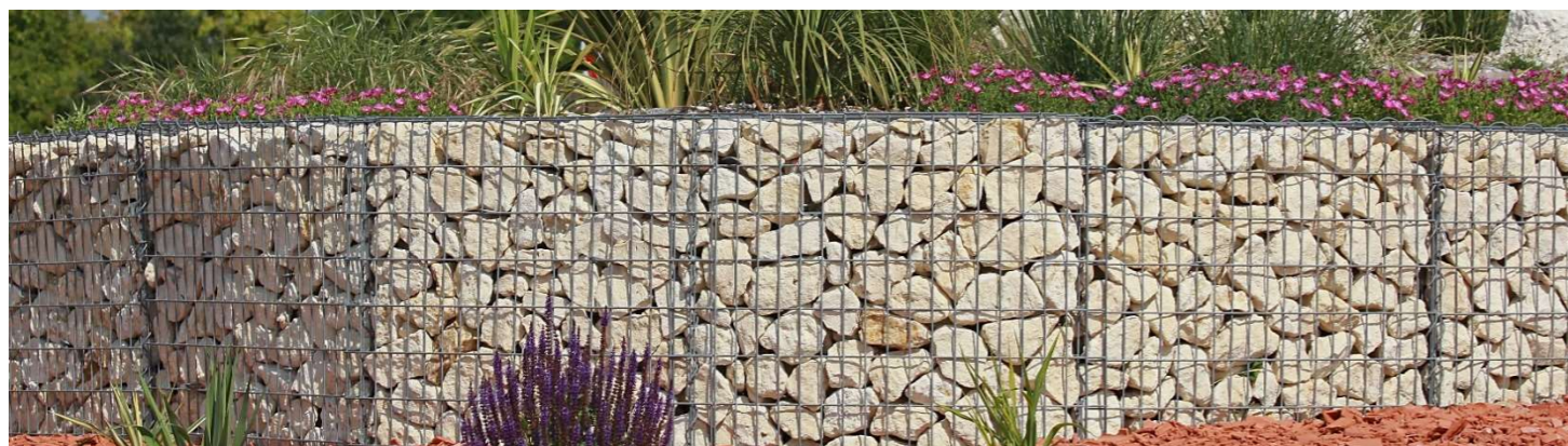
Reciklirani kamen, gabioni ,izvor: https://www.mainlandaggregates.co.uk/quarried-aggregates/quarried-gabion-stone.html
