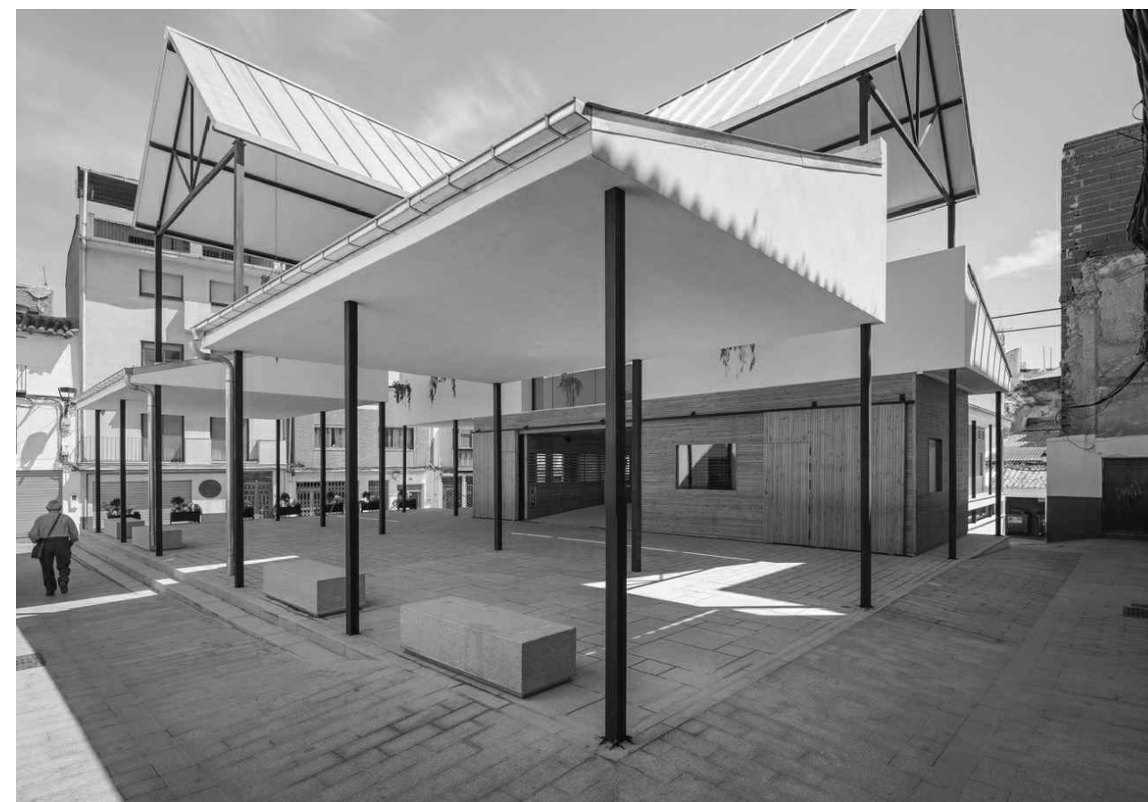
Municipal Food Market and Youth Center Rehabilitation/cÁcrono Arquitectura, Španjolska, 2019. g.
