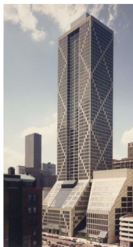
Slika 2.3.2.14 Onterie Center, Chicago, SAD, 1986.
