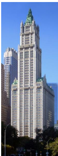
Slika 1.2.1.4 Woolworth Building, New York, 1930.
