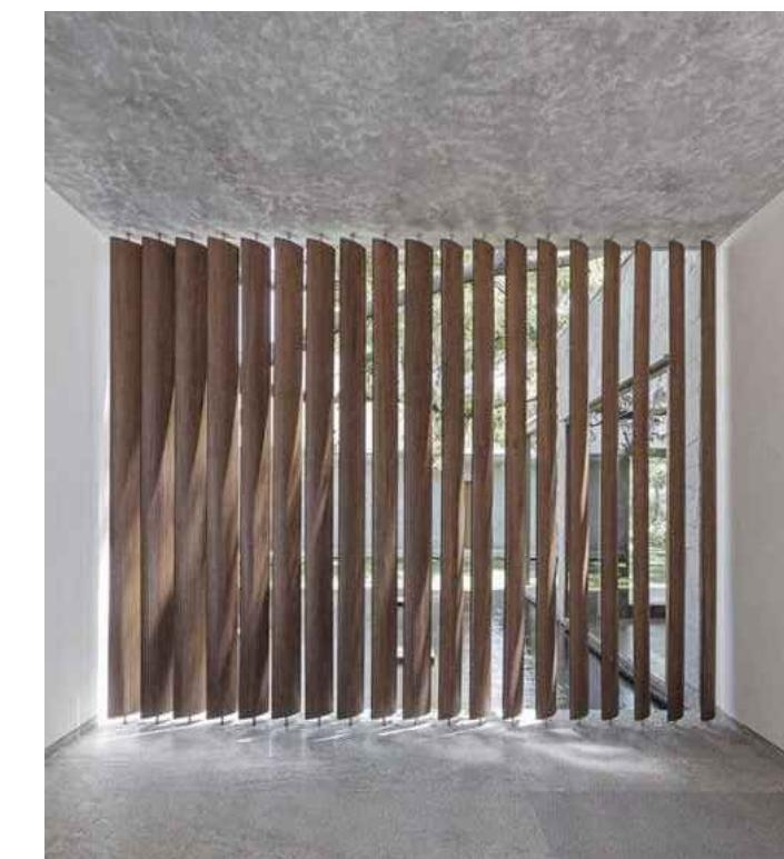
DRVENI ROTIRAJUĆI PANELI IMAJU DVJE ULOGE. PRVA ULOGA IM JE ZAŠTITA OD SUNCA, TE SAMOSTALNA MOGUĆNOST KONTROLIRANJA DOTOKA SVIJETLOSTI. DRUGA ULOGA IM JE U CILJU POSTIZANJA OSJEĆAJA SIGURNOSTI. PRILIKOM POTPUNOG OTVARANJA STAKLENE STIJENKE DRVENI PANELI ONEMOCUĆAVAJU PROLAZAK, TE SLUŽE U VIDU OGRADE, ALI ONO NAJBITNIJE MIJENJAJU POSTOJEĆE REŠETKE NA PROZORIMA SA HUMANIJIM PRISTUPOM.
