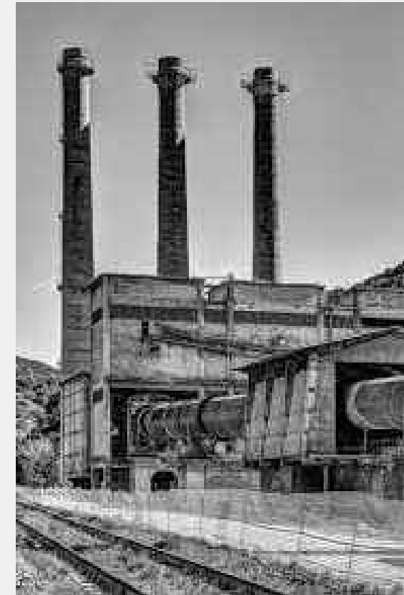
Akcenti u prostoru-tri dimnjaka [ https://encrypted-tbn0.gstatic.com/images?q=tbn:ANd9GcQOqegvOJKSWBy-0eSIRmsrgg2zHI_n886Ulw&usqp=CAU ]
