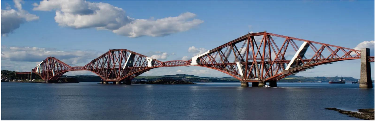
Figure 6. Forth bridge, Scotland
