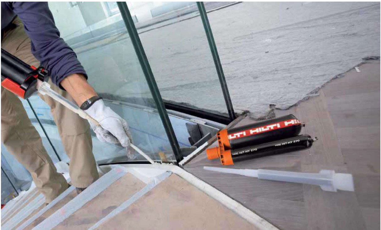
Figure 2.27 – Applying of HILTI ,HY-270 [5]
