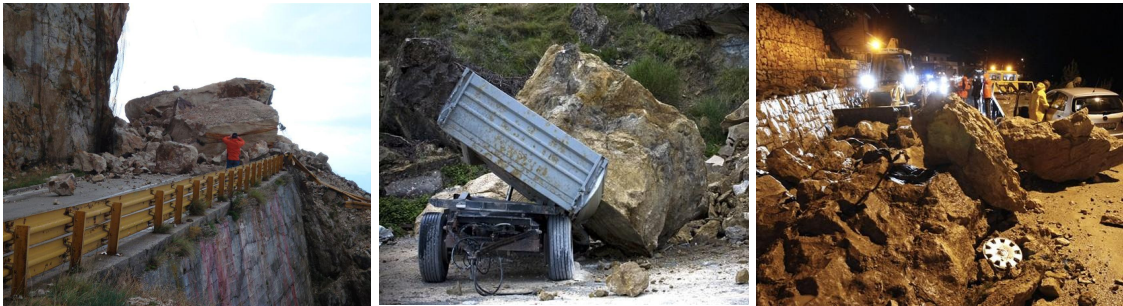
Figure 1.1: Rock falls hitting the coastal roads: Omiš, April 2012.; Omiš, April 2012.; Krilo Jesenice, March 2010.
