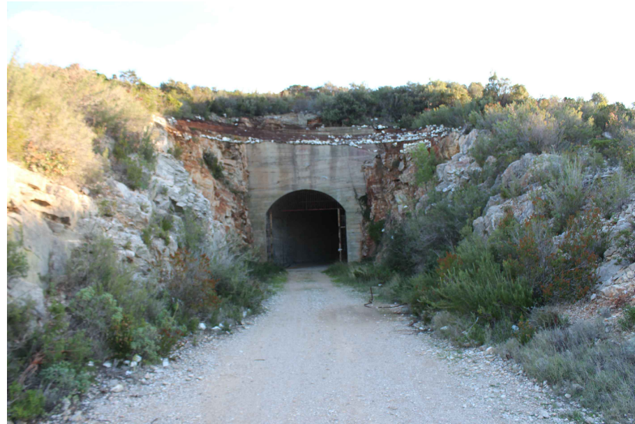
Ulaz u tunel
