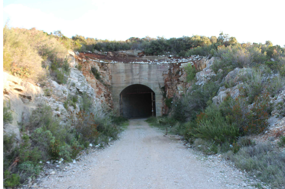
Ulaz u tunel
