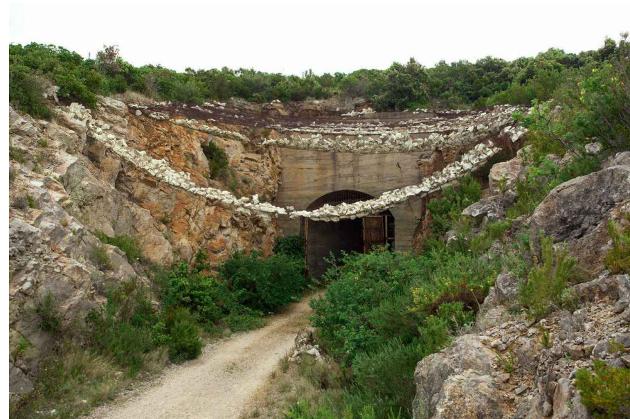
Podzemni tunel, Stupište
